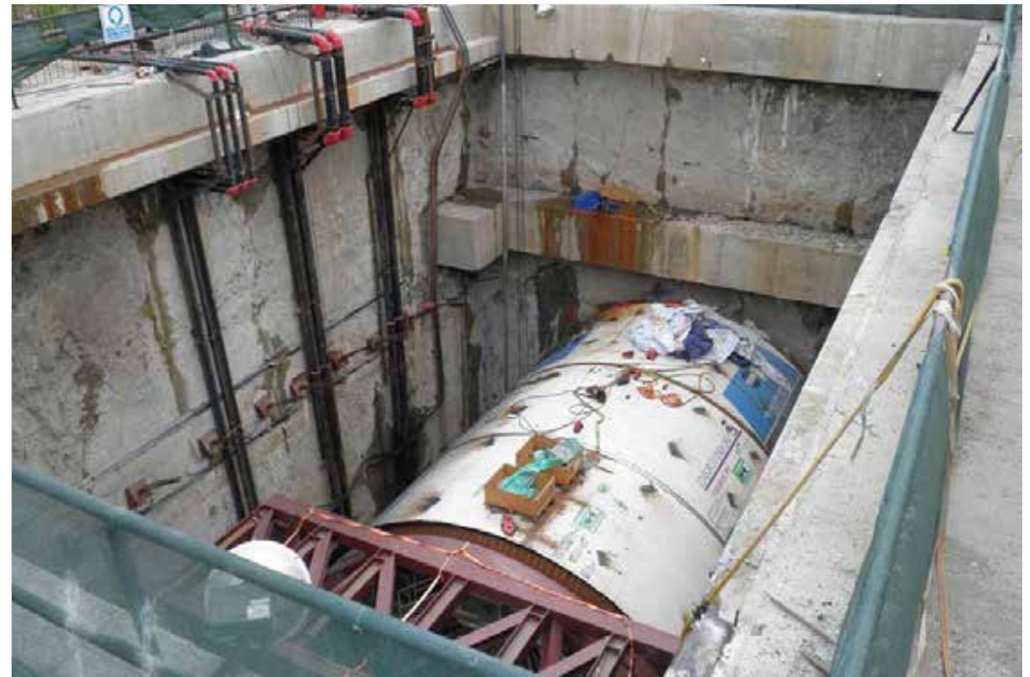
TBM Metro 1 Panama City - Panama
